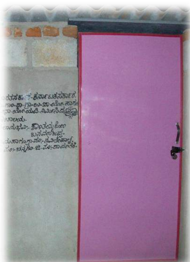
Picture 4 Completed toilet under Jaldi NBA
